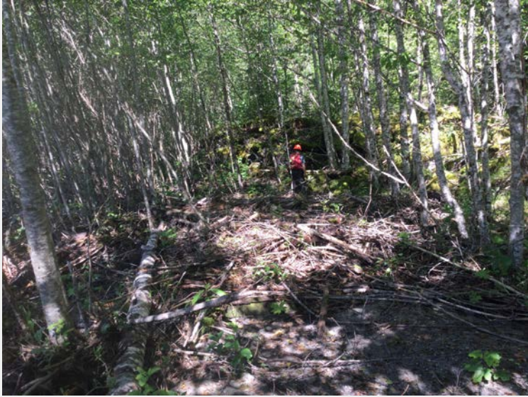
Old rock berm constructed within floodplain under vegetated cover
