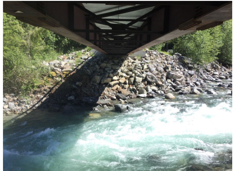
Right Bank Abutment when facing downstream
