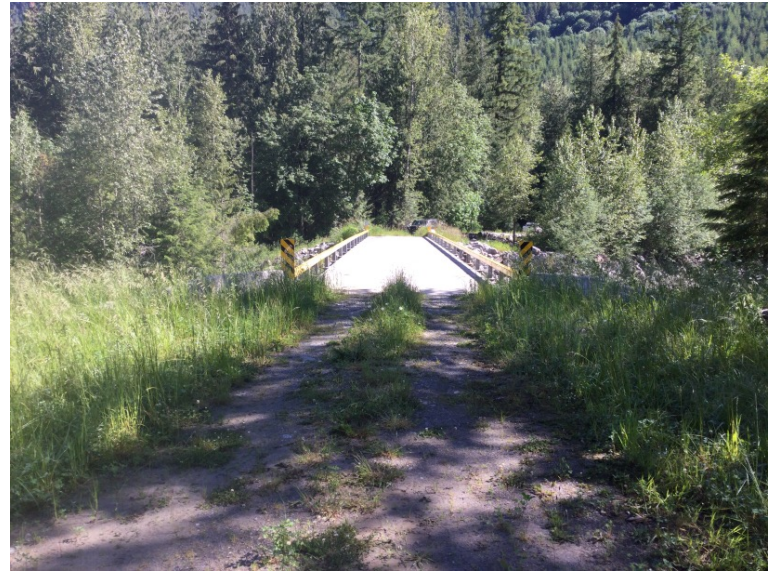
Approach from Left Bank when facing downstream
