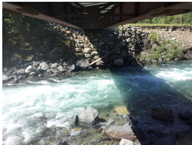
Left Bank Abutment when facing downstream
